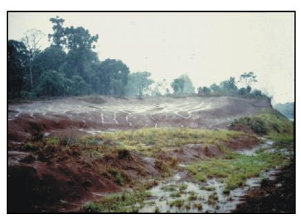
Fig. 5-2: Rill erosion an deposition at the foot of the slope after road construction. San Pedro, Misiones (Photo: M.F.Rau, 2001.
